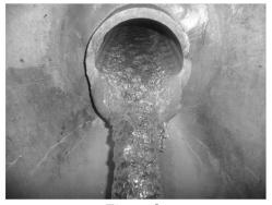
Figure 8. Carbonate incrustation in an inlet piping in shaft S64
