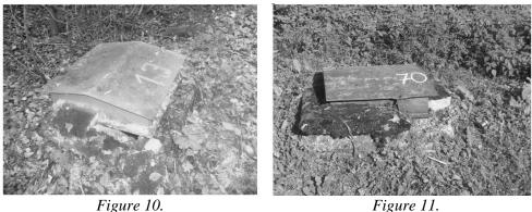
An example of destruction of concrete heading – shaft S20
