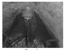
Figure 6. Roots in inlet piping of shaft S6
