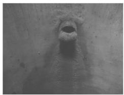
Figure 9. A clear reduction of piping crosssection as a result of incrustation (shaft S 117)
