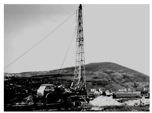
Figure 19. View of the drilling rig during the drilling of well G-4
