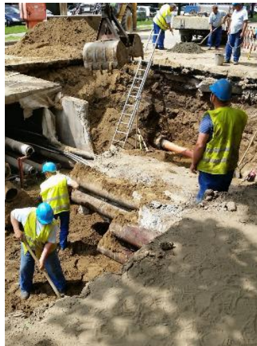
Figure 1. Repairing a burst pipe on a road (internet_5)
