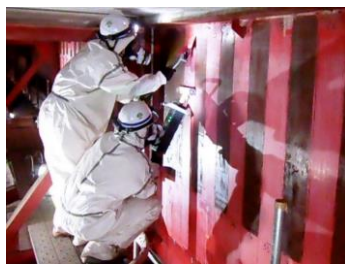
(a) Appearance of paint-coating removal
